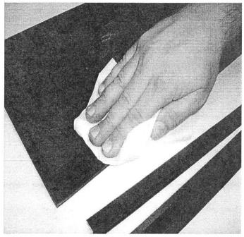
STEP 6: USE A DRY LINT FREE CLOTH TO WIPE DOWN THE SAME SECTION IN STEP 5... LET ALL AKTIVATED SURFACES DRY FOR 10 MINUTES MINUMUM
