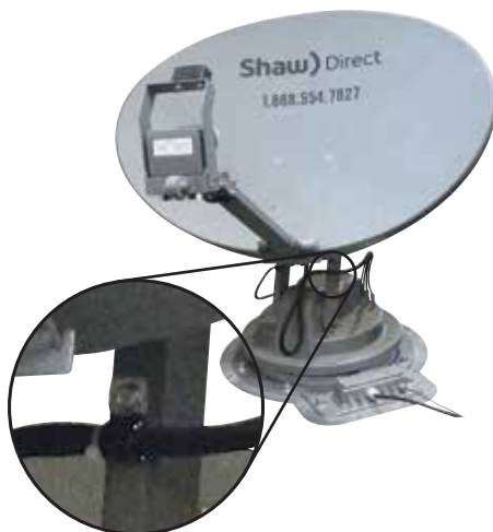
P-clamp installed 15" from ends of sheathed cables, next to zip tie on sheathed cables
