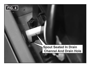
Seat spout into condensate drain channel and check to make sure the back edge of the spout is inside the drain hole. See FIG. 4.
