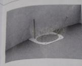
2 Use wedi template to mark cut out for drain body recess in subfloor.
