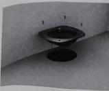
4 Recess wedi drain body and connect to ABS floor pipe using ABS cement glue. Fasten wedi drain pipe to subfloor using regular wedi wall panel screws. Over concrete floors adhere wedi drain body using wedi joint sealant instead.
