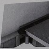
7 Make sure no thinset is pushed into the drain opening/area and that the gasket is firmly and entirely received in the drain body and in even position.
