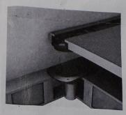
6 Install wedi base into thinset setting bed so that gasket on underside of base will safely drop into the drain body resting on the subfloor.
