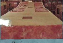
Roof A heavy plywood, center walkway and rear deck area are standard on a Kountry Aire. Rafters are heavy duty with 2 x 4 members every 16" Thick insulation gives a top blanket of comfort year around.
