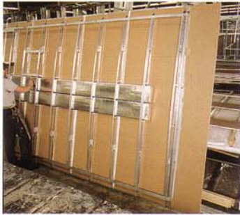
Truss-style rafters are built 16" on center and central air conditioning duct work is incorporated into the design to provide a more efficient central air conditioning system.
