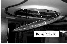
panel has released, let it swing gently down to rest on its retaining straps. You can snap the return air louvers down to access the filters.
