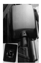
The vent installed in the bathroom is also powered by 12 volt electricity. This vent is controlled by the ON/OFF switch located on the wall. A vent similar to the one installed in the kitchen is optional.
