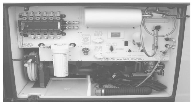
The heart of the plumbing in your King Aire is the exterior water compartment. All plumbing functions can be controlled from this location. Additionally, the connection points for city water, sewer rinse, and holding tank draining are all located in this compartment.
