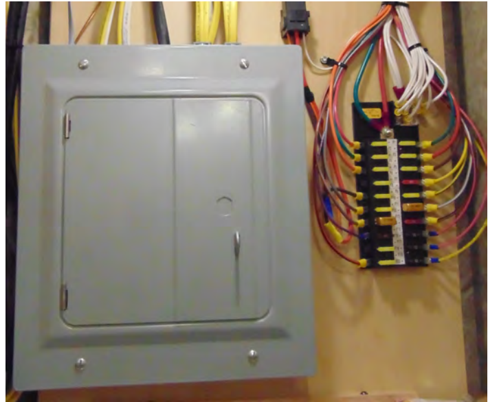
Class A House Fuse Panel Example
