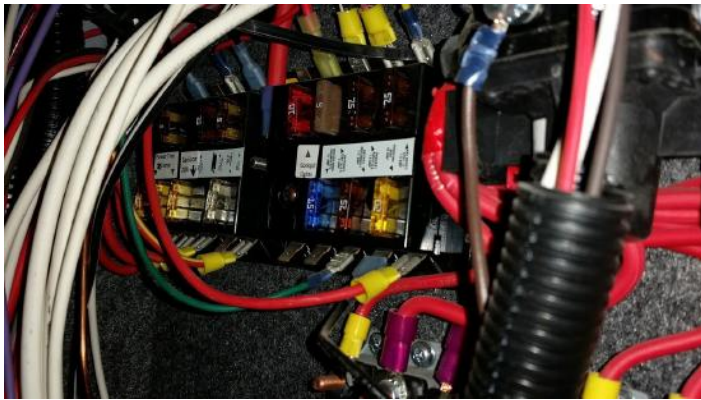
Sample: Cord Compartment Mini-Breakers
