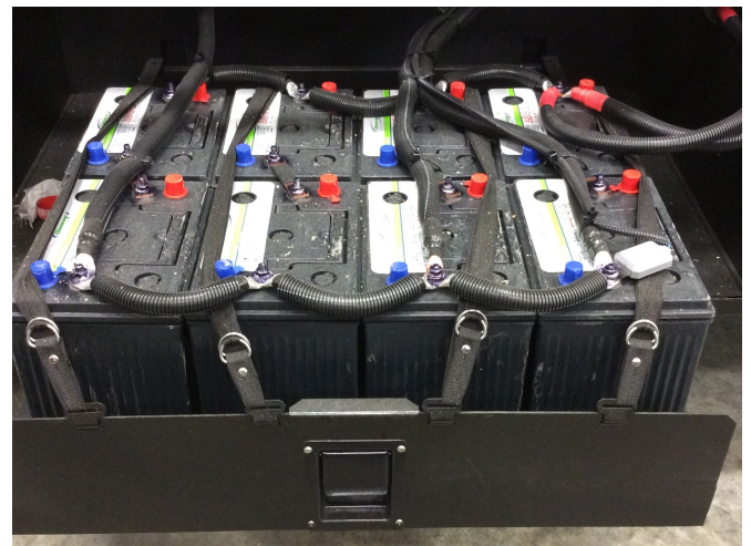
House Battery Bank Example
