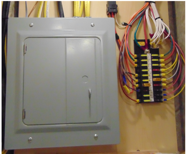
Class A House Fuse Panel Example
