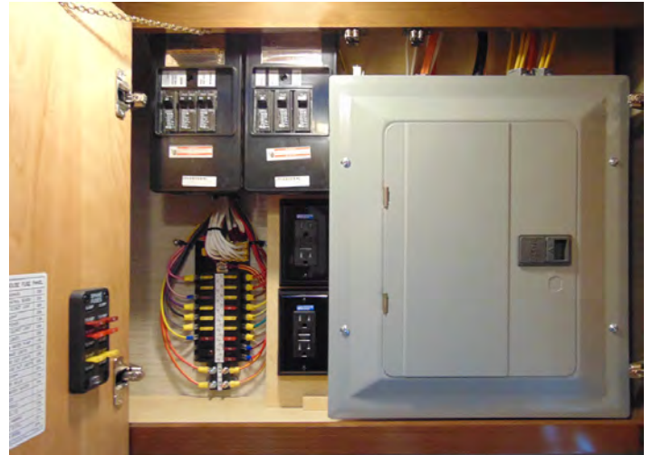
Diesel Pusher Fuse Panel Example
