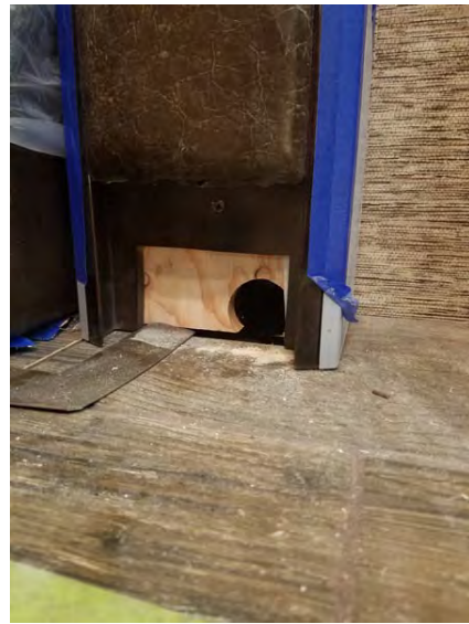
King Aire Access Point
