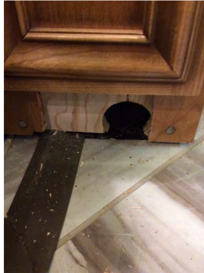
Mountain Aire Access Point
