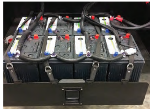
House Battery Bank Example
