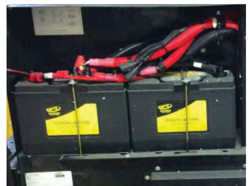
Chassis Battery Bank Example
