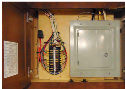
House Fuse Panel Example
