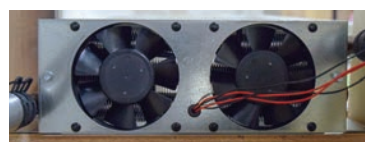
Oasis Dual Fan on Basement Heat Exchanger
