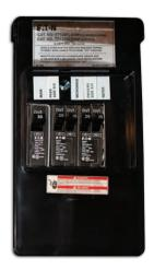
The subpanel is installed to limit the AC power use to specific circuits when the electricity is supplied by the inverter. Some inverters may be used to power a specific circuit. In this case, a subpanel is not used.
