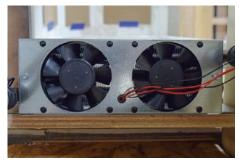
Oasis Dual Fan on Basement Heat Exchanger
