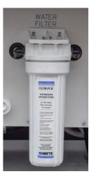
5. Reattach the canister to the filter housing by rotating the canister until it tight. Do not over tighten the canister when attaching it back to the housing.
