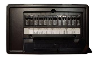
The EMS control module automatically senses the available power being supplied to the coach. The module determines whether it is connected to a 50 Amp (240 Volt) or the generator. On 120 Volt service, it is unable to determine if the source is providing 30, 20 or 15 Amp shore power. Depending on available power, it can control up to seven loads.
