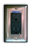
option, a separate GFCI is installed in the bathroom or near the main breaker box. Units with the holding tank heat pad option will have an additional GFCI located in the basement area; however, the exact location varies.
