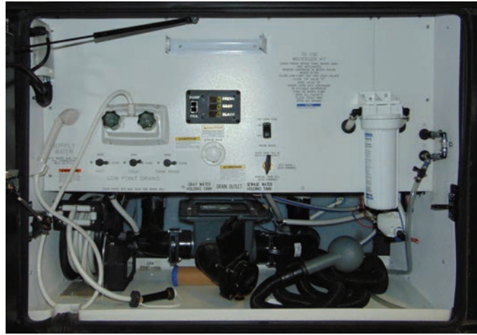
Mountain Aire Water Compartment
