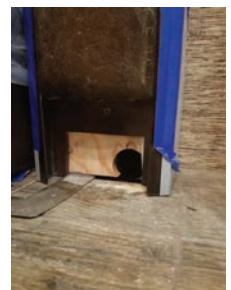
King Aire Access Point
