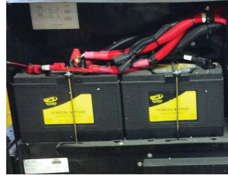
Chassis Battery Bank Example
