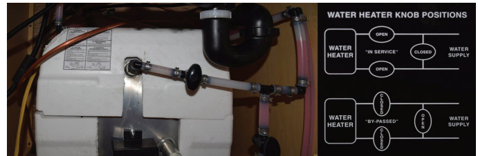
3 Bypass Valve System
