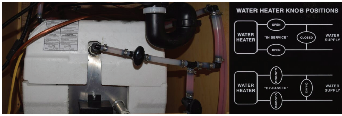
3 Bypass Valve System
