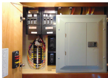
Diesel Pusher Fuse Panel Example
