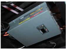
The LCD Screen changes depending on the operating mode of the inverter.
