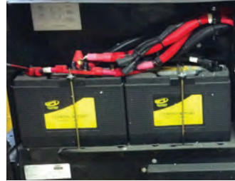
Chassis Battery Bank Example
