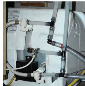
2 Bypass Valve System
