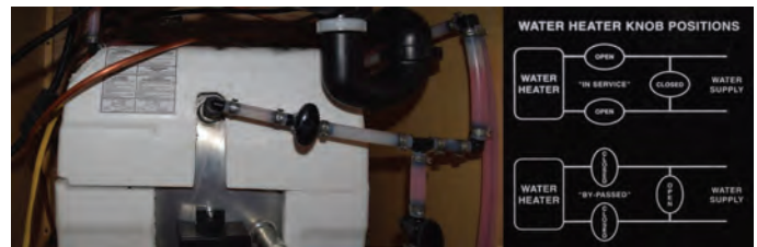
3 Bypass Valve System
