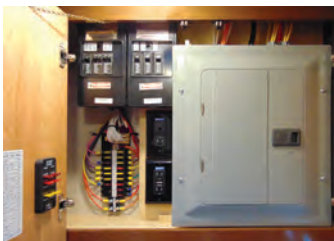
Diesel Pusher Fuse Panel Example
