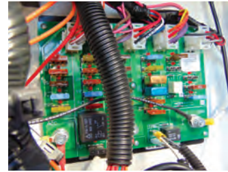
Example of a KIB Fuse Panel
