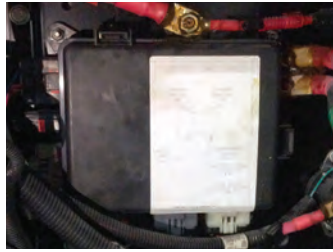
Freightliner Chassis Fuse Panel Example
