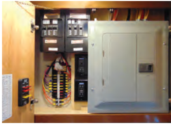
Diesel Pusher Fuse Panel Example
