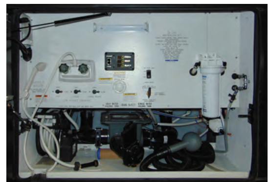
Mountain Aire Water Compartment
