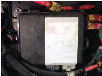
Freightliner Chassis Fuse Panel Example
