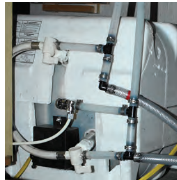
2 Bypass Valve System
