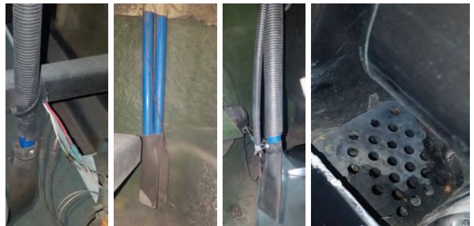
Roof Drain Catch Basin Strainer Examples
