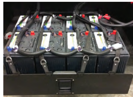
House Battery Bank Example
