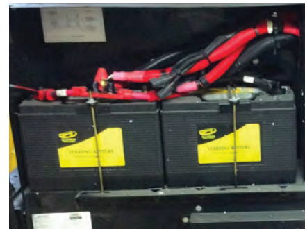
Chassis Battery Bank Example
