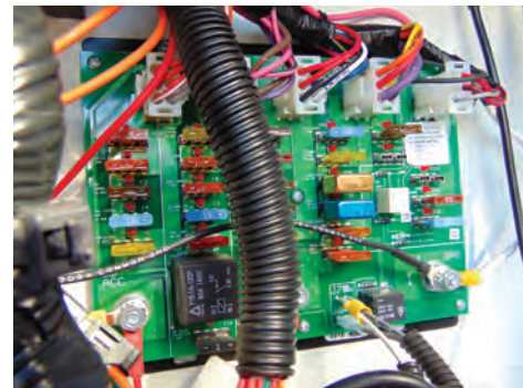
Example of a KIB Fuse Panel
