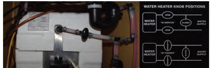
3 Bypass Valve System
