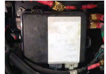
Freightliner Chassis Fuse Panel Example
