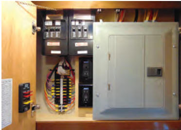
Diesel Pusher Fuse Panel Example
