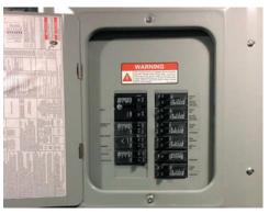
The breakers are resettable by simply flipping the breaker to the 'off' position, and then back to the 'on' position once the overload condition is removed. All 120 Volt circuit breakers are located in the main service panel unless the coach is equipped with an inverter/charger. These units are also equipped with a subpanel.
