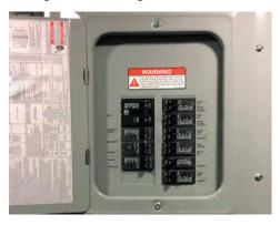
The breakers are resettable by simply flipping the breaker to the 'off' position, and then back to the 'on' position once the overload condition is removed. All 120 Volt circuit breakers are located in the main service panel unless the coach is equipped with an inverter/charger. These units are also equipped with a subpanel.
