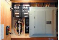
Diesel Pusher Fuse Panel Example
