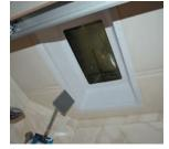
The skylight should be inspected with the roof and components, and the sealant should be maintained. Some sealants are not compatible with the skylight material. Newmar recommends using Surebond SB-140 butyl sealant around the skylight.
