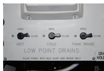
Low Point Drain Configuration Examples
