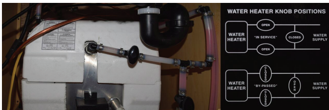
3 Bypass Valve System
