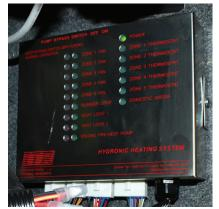
The Zone Control Board (Figure 8-5) contains seven green LED's for Power, Zone 1, 2, 3, 4 and 5 Thermostats, and Potable Water.
