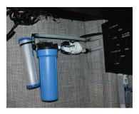
range, to provide pathogen reduction without the use of harmful chemicals or heavy metals. Use of LEDs allows the PearlAqua Micro to achieve full intensity power upon start-up, withstand unlimited power cycles without impacting device life, and eliminate disposal processes.
