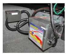
Newmar currently uses three sizes of converters: 45, 60, and 80 Amp models. Previous units may have a 55 or 75 Amp converter or two 45 Amp converters with a total of 90 Amps available. When replacing a converter, it is necessary to use the same size converter to ensure sufficient wiring and breakers for the converter's input and output ratings.
