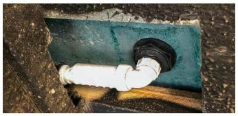
Foreign objects, such as hair, in the trap may allow odor to enter the coach and impede or slow water drainage and require occasional cleaning. When removing the waterless trap for cleaning, the ridges must be down and the direction of water flow must be correct when re-installed.
