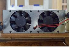
Oasis Dual Fan on Basement Heat Exchanger
