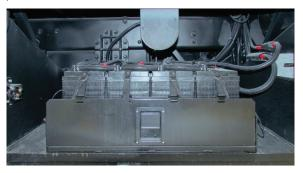
Any time one battery is replaced, it is important to test the rest of the batteries in the system to make sure they are still functioning properly and efficiently. If one defective battery is replaced, while leaving another weak or defective battery, lowered performance, or ultimately damaging the new or good batteries, may result.
