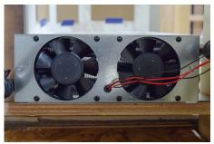
Oasis Dual Fan on Basement Heat Exchanger
