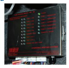
The Zone Control Board (Figure 8-5) contains seven green LED's for Power, Zone 1, 2, 3, 4 and 5 Thermostats, and Potable Water.
