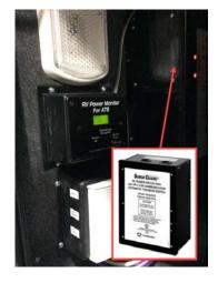
If there is no error message and the display instead reads "Delay Active" this means that the fault condition has cleared and that the switch is going through a 2.5 minute delay before it will attempt to close the contactor again. Wait until this delay is over to see if the ATS correctly closes its contactor.
