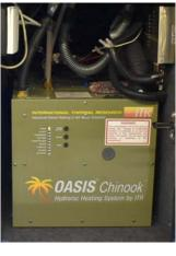
Zone 1, 2, 3, 4, 5 Fans, Summer Loop, Heat Loop 1, Heat Loop 2, Engine Pre-heat Pump Paired LED's (Red/Green): The nine paired LED's indicate the functionality of the corresponding devices. The green LED will turn ON when the device is operating normally. The red LED turns ON if a fuse has been blown.
