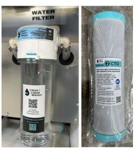
Change the filter at least every six months and at any time you notice decreased water flow or notice an unpleasant taste, odor, or algae after flushing and sanitizing the water system. Water filters and fresh water system maintenance are the customer's responsibility to ensure safe potable water.
