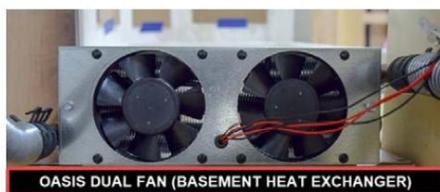
OASIS DUAL FAN (BASEMENT HEAT EXCHANGER)
