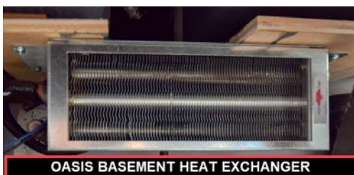
OASIS DUAL FAN (BASEMENT HEAT EXCHANGER)
