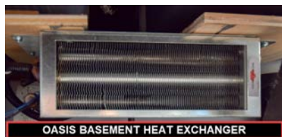
OASIS BASEMENT HEAT EXCHANGER
