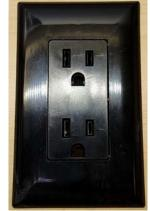
Do not use an adapter, cheater, or extension cord that breaks the continuity of the ground circuit to the ground pin. Never remove the ground pin from a plug in order to connect it to a two-pronged ungrounded outlet.
