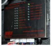
Loop 1 pump. When Zones 3, 4, and 5 are calling for heat, the zone control board will activate the Heat Loop 2 pump.
