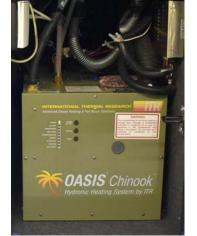
For the Zone Control Board to respond to a call for heat, the coolant temperature inside the Oasis® Chinook must be above 120F.
