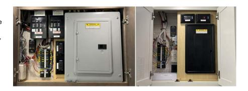
Some external components are fused in the house fuse panel. For example, the fuses for the water pump, water heater, security lights, and basement storage lights may be located in this panel.
