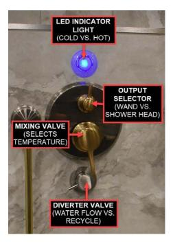
Once the water is warm, the system's LED indicator light will let the user know when it is time to adjust the diverter in order to allow water to freely flow from the shower. If you use the diverter valve to stop water flow during the shower once the indicator light turns red, you are diverting hot water to the fresh tank.
