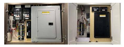
This panel contains fuses and breakers that are connected to the main appliances in the coach, from the refrigerator and television to the lights in the bedroom and slideouts.
