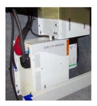
On units equipped with an EMS, the subpanel is located in the same breaker box but is separated in the interior of the main panel. The coach battery bank supplies the inverter 12 Volt power and has a high amp fuse link on the positive lead from the batteries and is located near the battery bank.
