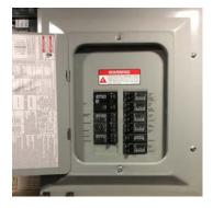
The breakers are resettable by simply flipping the breaker to the 'off' position, and then back to the 'on' position once the overload condition is removed. All 120 Volt circuit breakers are located in the main service panel unless the coach is equipped with an inverter/charger. These units are also equipped with a subpanel.
