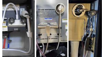
The faucet operates just as it would in the kitchen or bathroom. When finished using the exterior shower, shut off both the hot and cold valves. Do not simply shut off the valve on the shower head itself, as it may cause hot and cold water to mix at the exterior shower and could allow drastic changes in water temperature throughout the coach.
