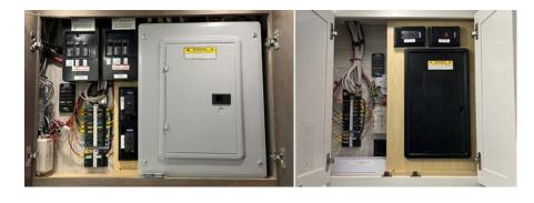
Some external components are fused in the house fuse panel. For example, the fuses for the water pump, water heater, security lights, and basement storage lights may be located in this panel.
