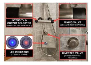
valve to stop water flow during the shower once the indicator light turns red, you are diverting hot water to the fresh tank.
