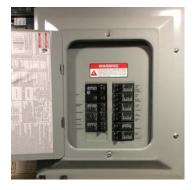
The breakers are resettable by simply flipping the breaker to the 'off' position, and then back to the 'on' position once the overload condition is removed. All 120 Volt circuit breakers are located in the main service panel unless the coach is equipped with an inverter/charger. These units are also equipped with a subpanel.
