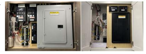
House battery and disconnect fuses are located in the compartment with the shore power cord. These fuses control the battery boost, battery disconnect, keyless entry, hydronic heat, LP detector, and entrance steps. In this same location, 12 volt circuit breakers provide power to the house fuse panel, slideout motors, power awnings, and the entry step.
