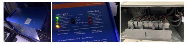
In this example, only the charger is on, and it is float-charging the house batteries.
