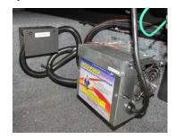
When replacing a converter, it is necessary to use the same size converter to ensure sufficient wiring and breakers for the converter's input and output ratings.
