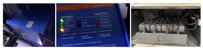
In this example, only the charger is on, and it is float-charging the house batteries.
