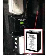
If no display is available, check the level of the input voltage to ensure it is within the proper operating limits. Also check that the ATS is correctly connected to chassis ground and that the neutral conductor is correctly connected to ground at the power pedestal. Wait 2.5 minutes to check if the fault condition was temporary and has cleared. If so, the contactor will pull in at the end of the 2.5 minute period.
