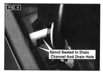
5. Seat spout into condensate drain channel and check to make sure the back edge of the spout is inside the drain hole. See FIG. 4.
